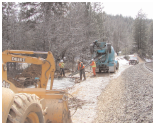
Upgrading Old Pipelines in Zone 3 PCWA maintenance crews in early April repaired a leaking section of the Gold Run Pipeline near the railroad tracks in Gold Run, above. A section of failed Techite pipe on the Secret Town Pipeline is pictured, below.
