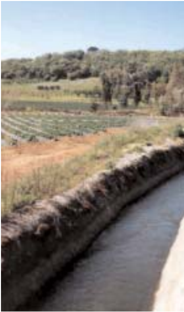
Gunite lining can reduce loss and make more water available to customers.
